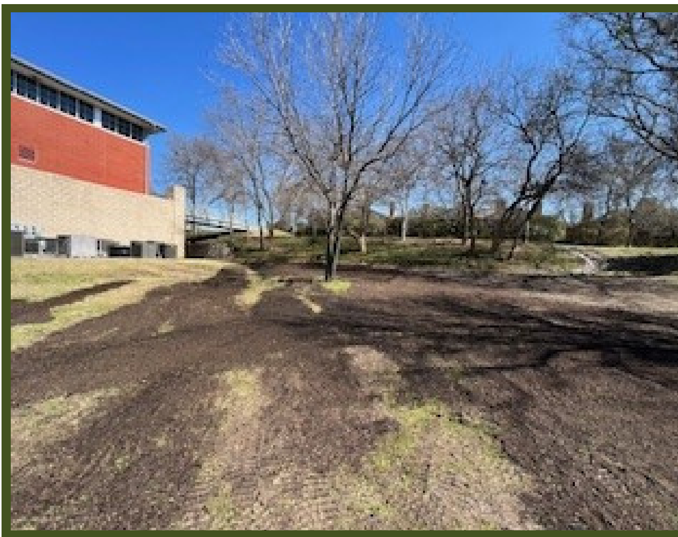
CITY HALL TURF INSTALLATION
