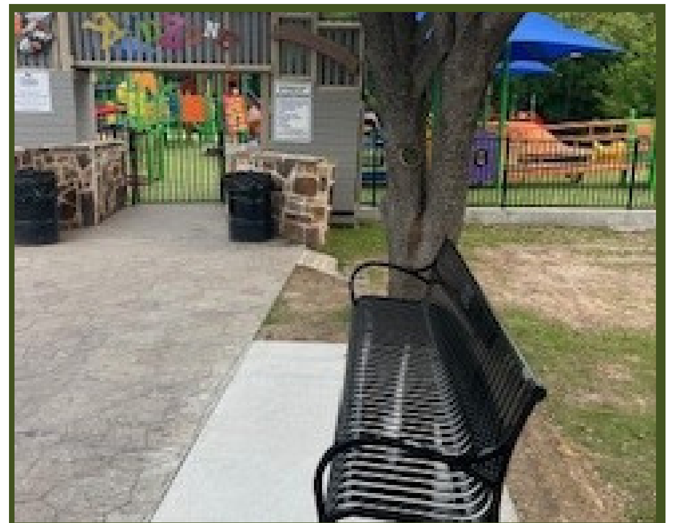
HARRY MYERS KIDZONE MEMORIAL BENCH INSTALLATION
