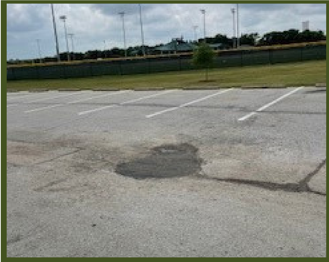
TUTTLE PARKING LOT REPAIR
