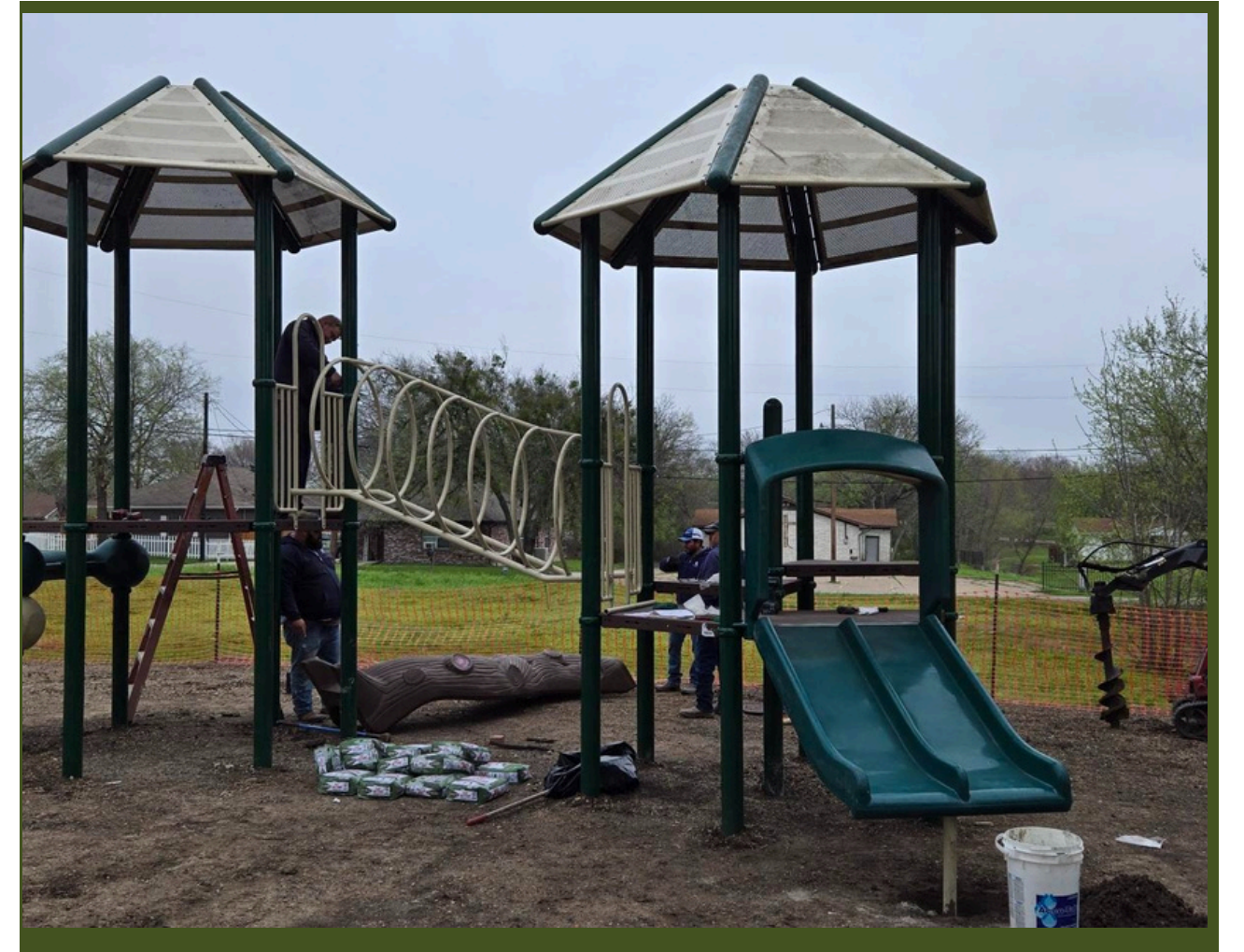
GLORIA WILIAMS PLAYGROUND SOD INSTALLATION
